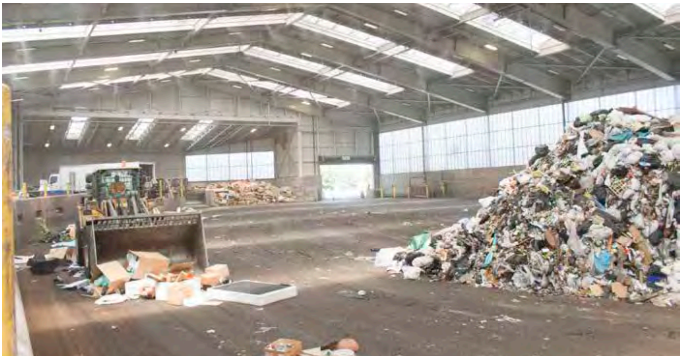
Bow Lake Recycling and Transfer Station
